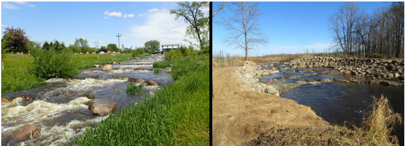
Rock Arch Rapids similar to the proposal – proposal will be smaller in scale than each above.
